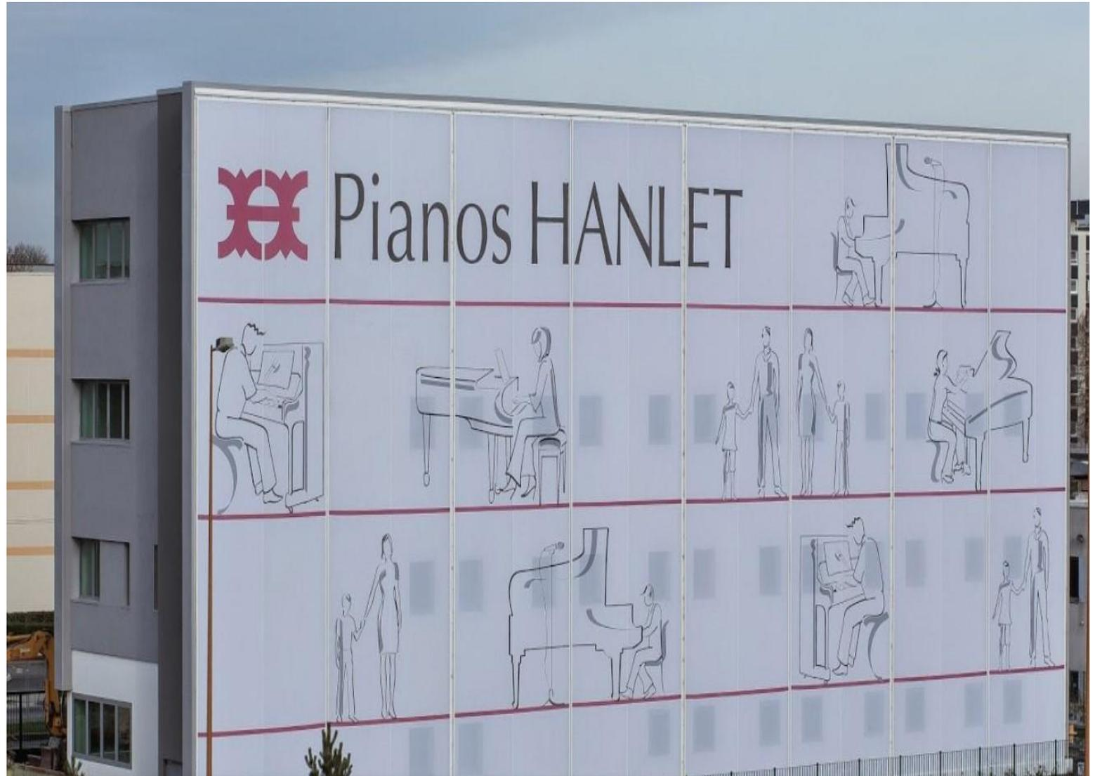
Textile facades are made of tensioning net fabrics.
