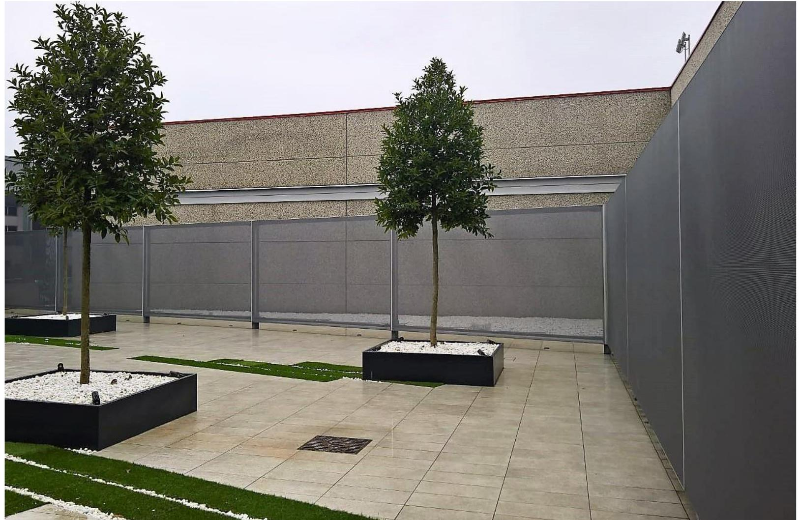
The textile façade is made with a micro-perforated material, available with different opening degrees. The façade is designed and made with fabrics and materials that will last more than 20 years.
